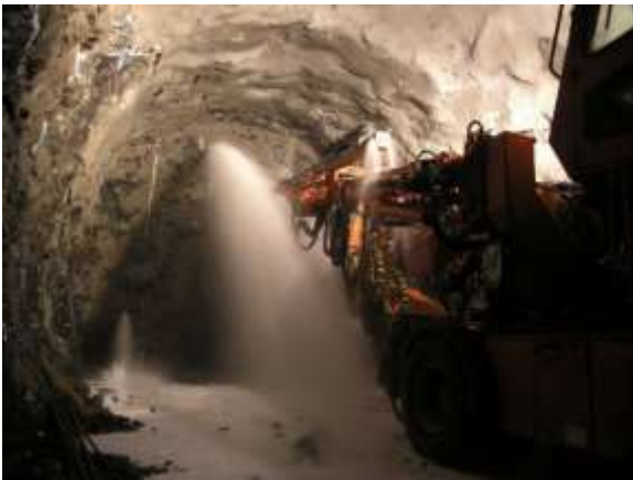
Figure 27. Water inflow into the Héðinfjörður tunnel. Figure courtesy of B. A. Harðarson.
