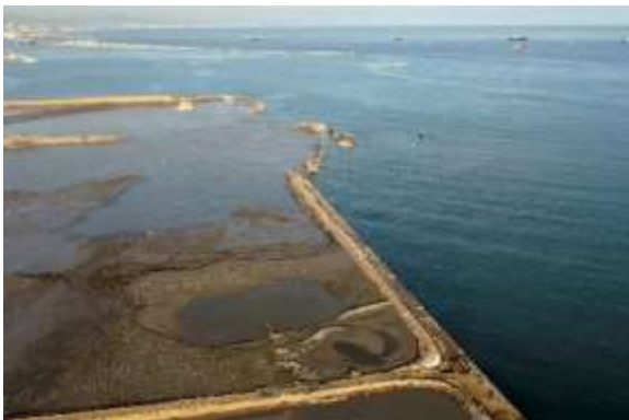
Figure 32. View of the Prat quay failed section
