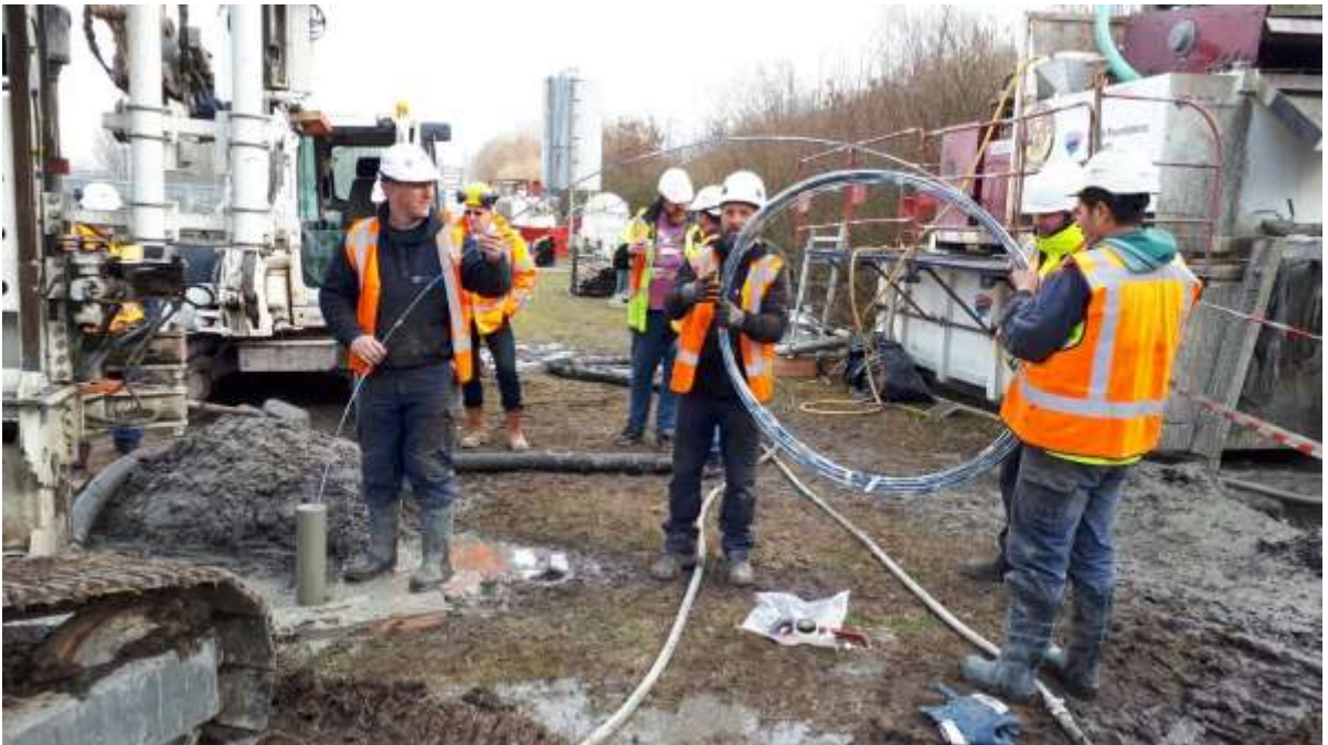
Figure 22. Installation of the instrumentation in a 67m deep micropile
