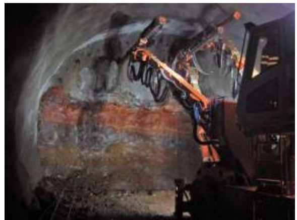
Figure 26. Drilling into a layered face at the Óshlíð road tunnel. Figure courtesy of B. A. Harðarson.
