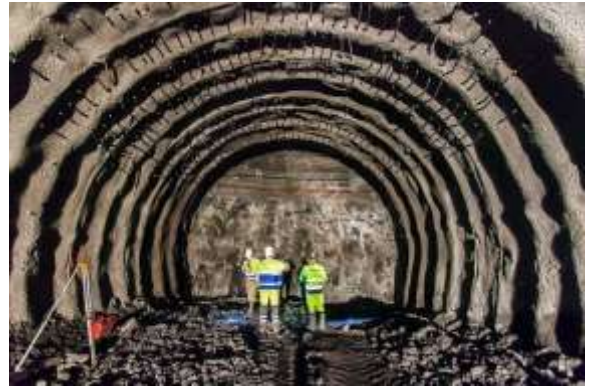
Figure 25. Lattice girders as a support in the 2-lane Vaðlaheiði road tunnel. Figure courtesy of B. A. Harðarson.
