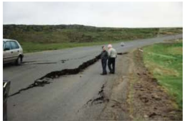
Figure 14. A pavement structure resting on a peaty subgrade in Holt, South Iceland that liquefied in the June 17, 2000 earthquake ( M_w 6.5). Figure courtesy of V. A. Ingólfsson.
