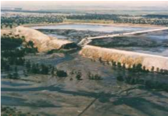
Figure 25. View of Aznalcóllar dam after failure
