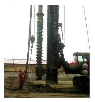
Figure 12. Screw pile with oversized portion of excavation auger at the bottom (Bottiau, 2014)
