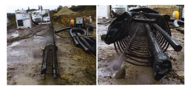
Figure 14. Haren test site - Illustration of the reinforcement cage provide with reservation tubes for the extensometer system
