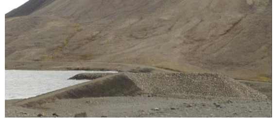
Figure 5. Fuse plug at Hágöngulón reservoir. Rock-fill dikes upstream and downstream from the saddle dam. Photo: Kristín Martha Hákonardóttir
