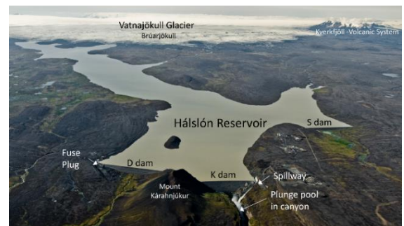
Figure 4. The Hálslón reservoir, dams, spillway and fuse plug (Sigtryggdóttir et al., 2016). Photo: Emil Thor.
