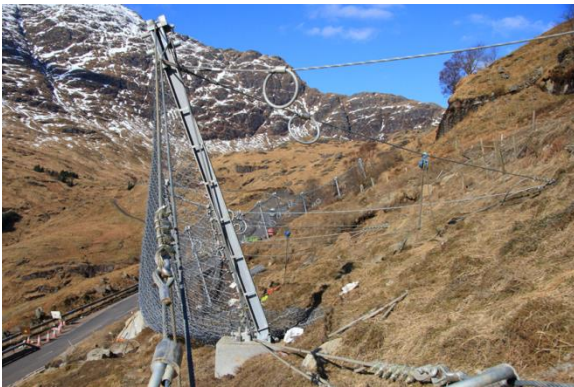
Figure 24. A33 Rest and be Thankful flexible debris fence.
