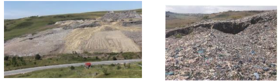
Figure 7. Example 5 – old landfill – major landslide - failure within waste mass
