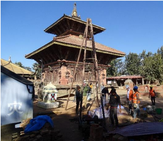
Figure 3. Drilling operation at Changu Narayan
