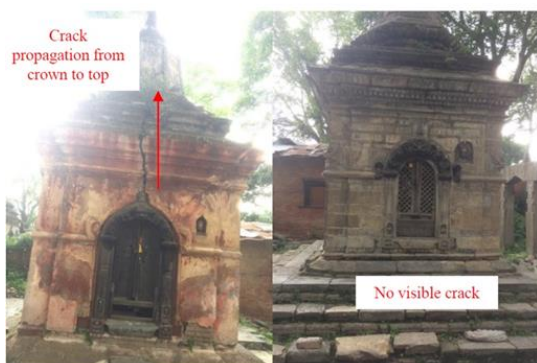
Figure 11 View of visible crack in a temple made of brick masonry and no such crack in a stone temple.
