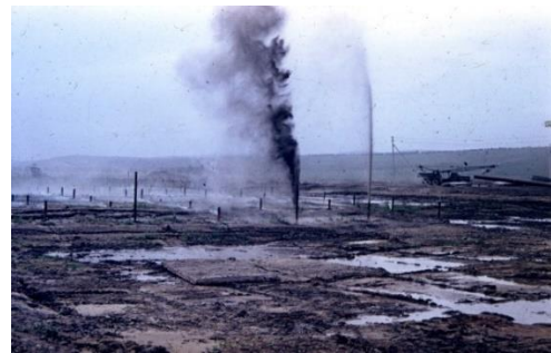
Figure 1. Compaction of loessial subsiding soils by hydroblasting method
