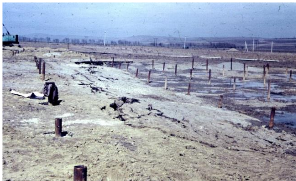
Figure 4. Site general view after soil compaction by hydroblasting method
