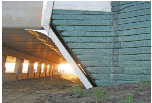
Figure 7. Executed overstep GRS Wall in the function as bridge approach and earth pressure relief to protect slender concrete wing walls of an ecoduct
