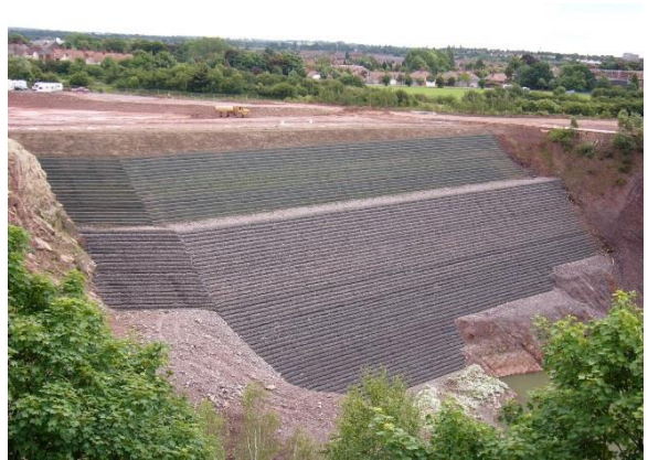
Figure 1. GRS wall after completion of construction
