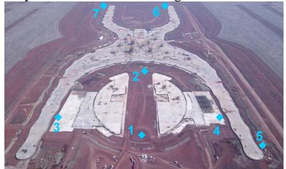
Figure 3. Pile test locations. The PTB sits on the X shaped raft and the GTC on the round raft.
