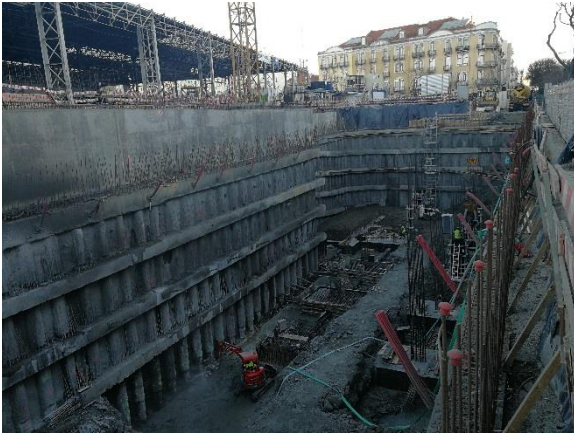
Figure 8. View of the final excavation works.
