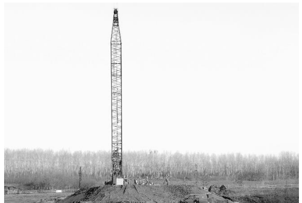
Figure 2. Test site and used crawler crane in the field investigation.
