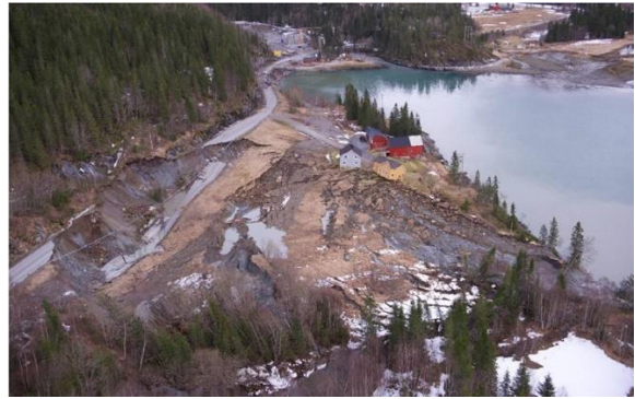
Figure 1. Overview. The first slide, Bjørnstokkvika and the power plant in the back, the second slide Bekkevold, in the front. Foto: Jørn Horn.
