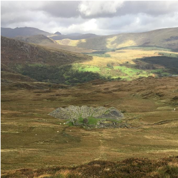
Figure 4 Radial spoil mound adjacent to an air shaft at Ffestiniog tunnel..
