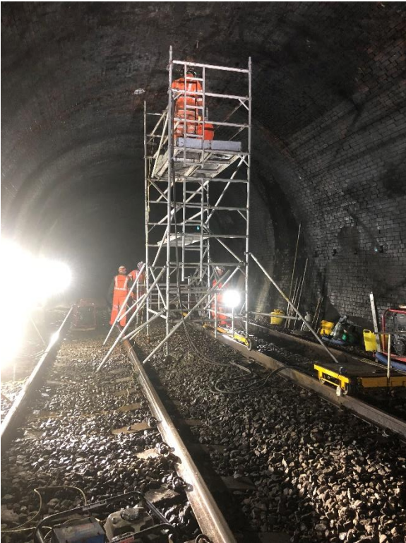
Figure 7 – Drilling coreholes into the tunnel roof of Lonlas Tunnel
