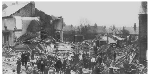
Figure 1 Clifton Hall Tunnel Shaft Collapse (Salford Voice 2017)
