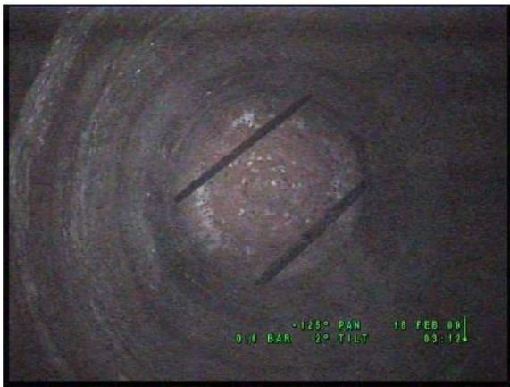
Figure 10 – CCTV inside Hidden Shaft on LNW Route
