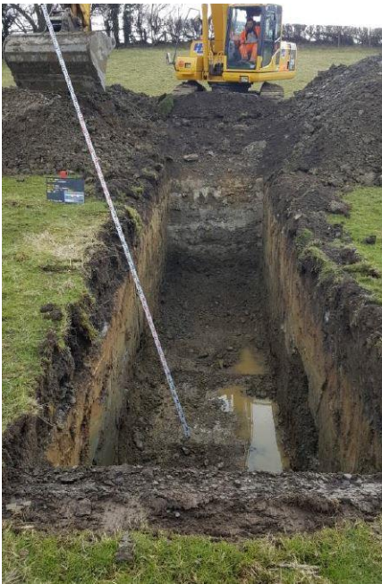
Figure 6 – Trial Trenching investigation (AMEY)
