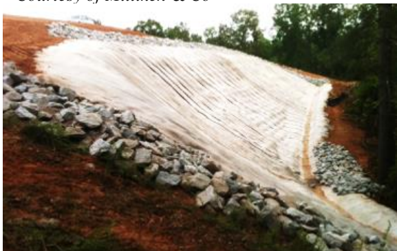
Figure 6. Completed GCCM facing with toe drain. Courtesy of Milliken & Co
