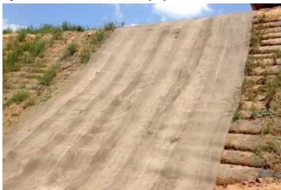
Figure 5. GCCM installation over wrap faced RSS. Courtesy of Milliken & Co
