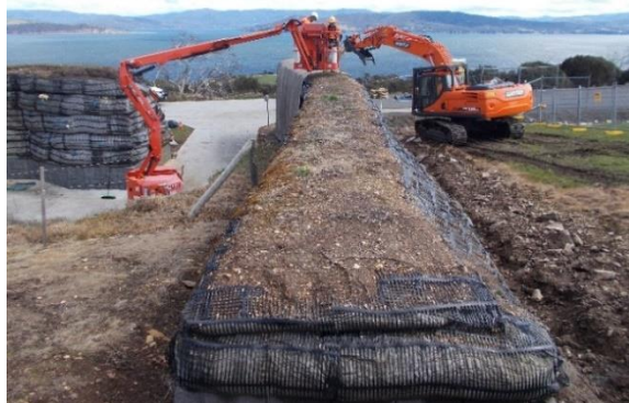
Figure 7. Wrap faced bund requiring permanent protection. Courtesy of Concrete Canvas Ltd.
