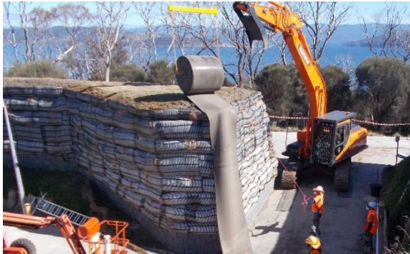
Figure 8. Placing GCCM to protect bund structure. Courtesy of Concrete Canvas Ltd.
