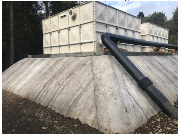
Figure 12. Completed RSS faced with GCCM.. Courtesy of Concrete Canvas Ltd.
