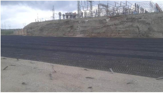
Figure 7: Load transfer platform construction
