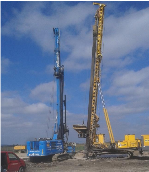
Figure 5: Subsoil improvement by stone columns
