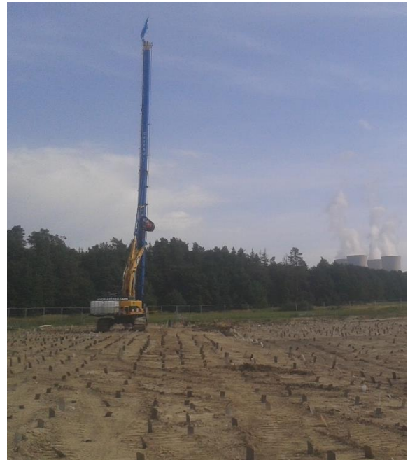
Figure 6: Subsoil improvement by prefabricated vertical drains
