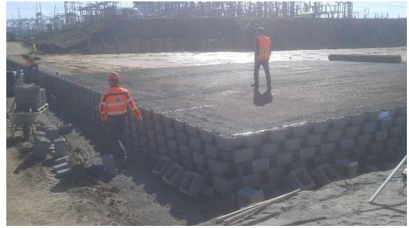
Figure 8: Reinforced soil retaining wall construction
