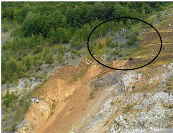
(a) before slope failure
