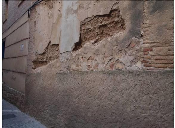
*Figure 1: Rising damp and delamination of cement render exposing the RE beneath, Tarazona city.*
