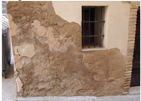
Figure 4: Surface delamination due to rising damp with salts efflorescence, Borja.
