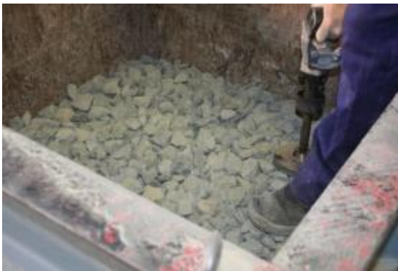
Figure 4 Preparation of ballast layer with a dynamic compactor
