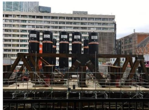
Figure 4: Test pile reaction frame with bentonite silos in the background (also used as ballast during the test)
