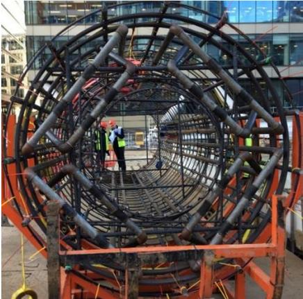
Figure 3. Pile cage with base grouting tubes shown
