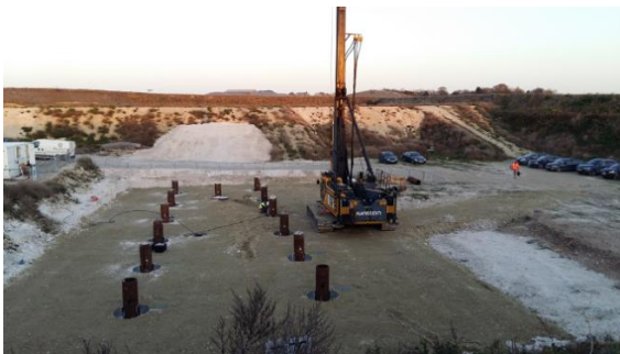
Figure 4 Piling operations underway at St Nicholas-at-Wade for ALPACA JIP programme;
