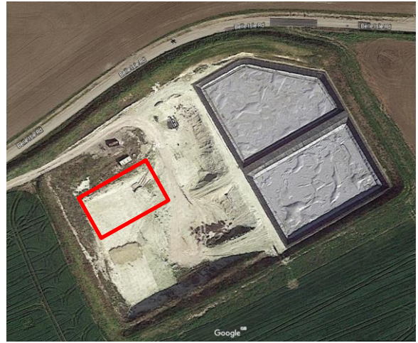
Figure 3 Aerial view from Google Earth of St Nicholas-at-Wade test site showing approximate test area for ALPACA JIP programme.
