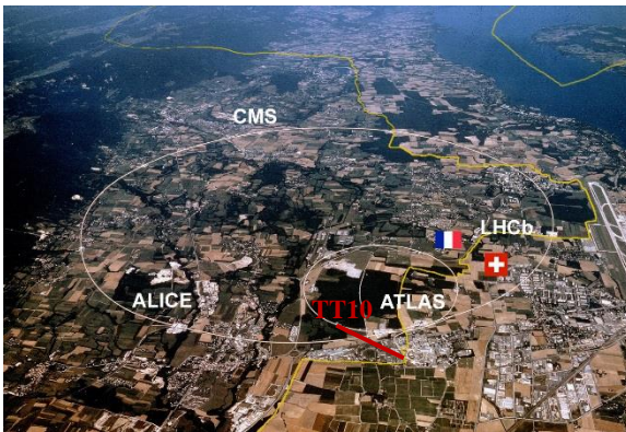
Figure 2. TT10 transfer tunnel location.
